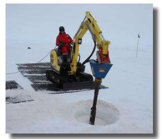
*Fig. 3.1.1.8: Drilling a 90 cm diameter hole. Larger holes need to be created by overlapping several holes.*
